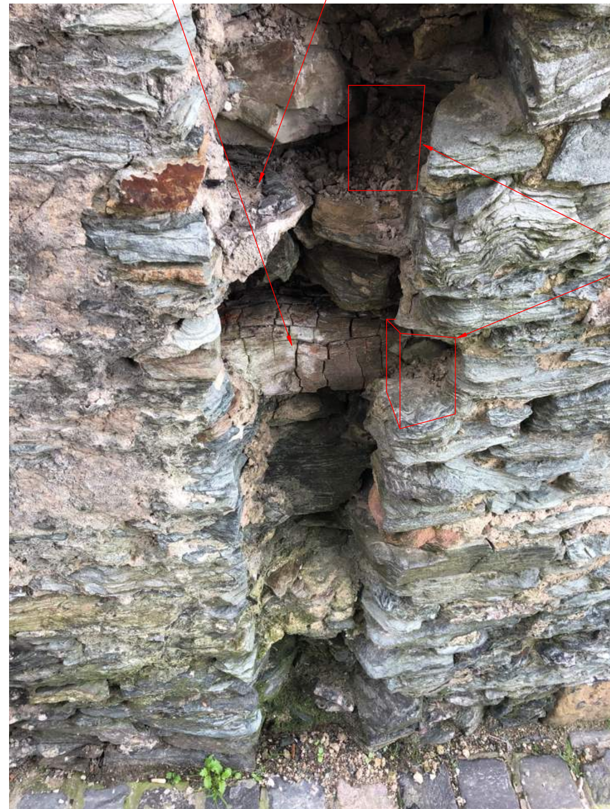
VIEW ON TYPICAL REBATE (SIMILAR ON 4 FACES)
