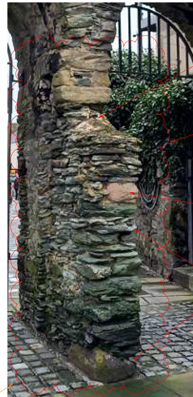
VIEW ON PIER FROM NORTH
