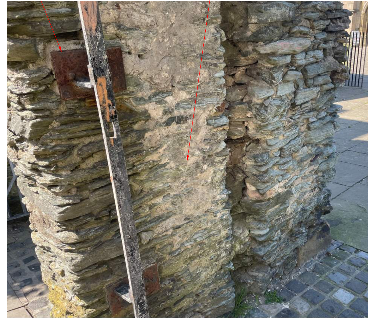
VIEW ON PIER FROM SOUTH
