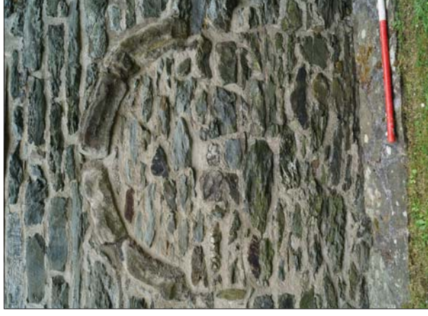
Plate 18. Detailed Shot of West Facing Gable
