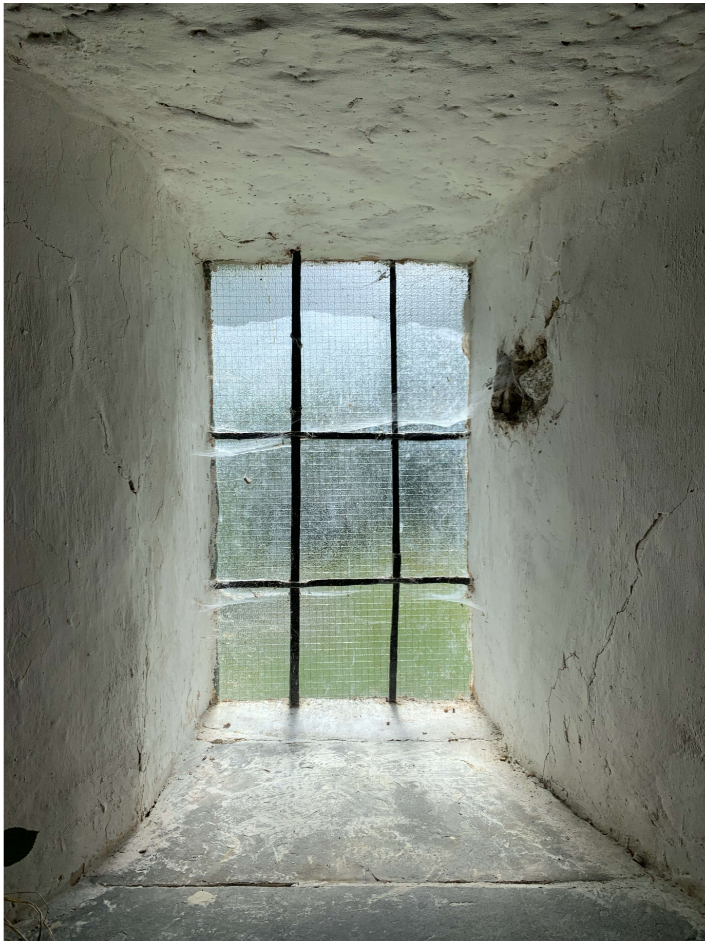
Window s11 as existing, internally.
