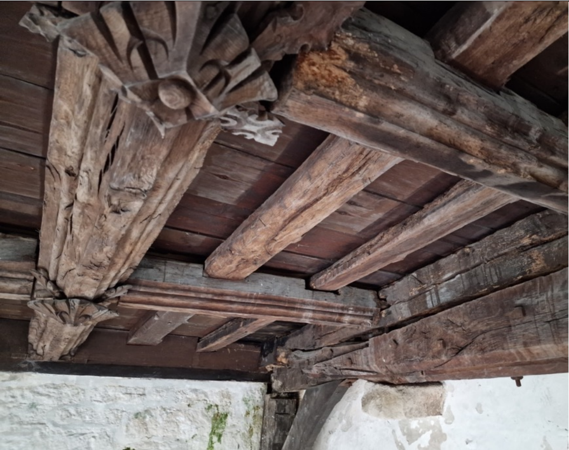
b Purlin connection (wider view, looking to south-west corner).
