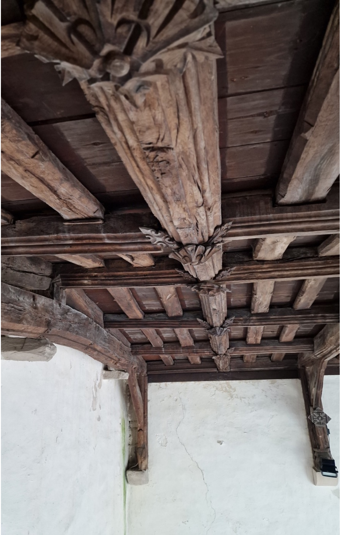
17 Timber ceiling bosses, purlins and upright post – view looking to the north-west corner of the nave.
