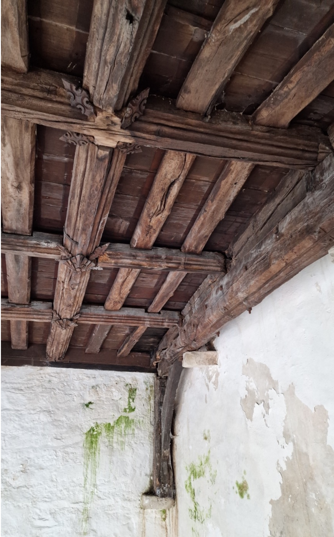
15 Timber ceiling bosses, purlins and upright post – view looking to the south-west corner of the nave.
