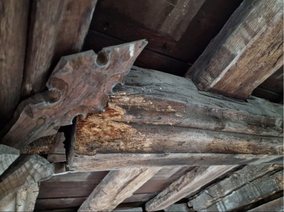
16 Purlin connection (detail).
