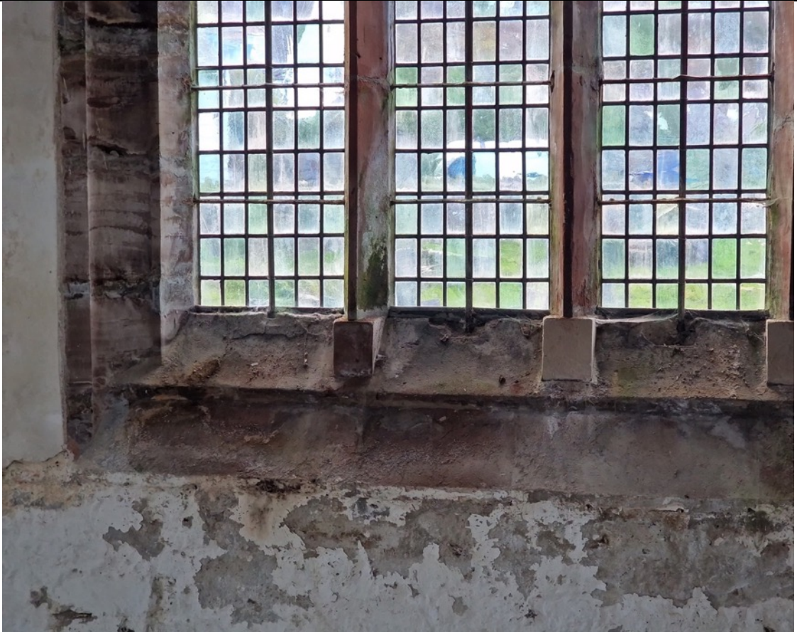
7. Window W05 from lift – Detail: Cill and base of mullions (internal view)
