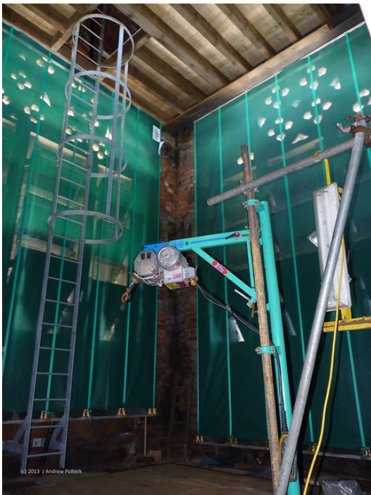
Image of the galebreakers during installation.
