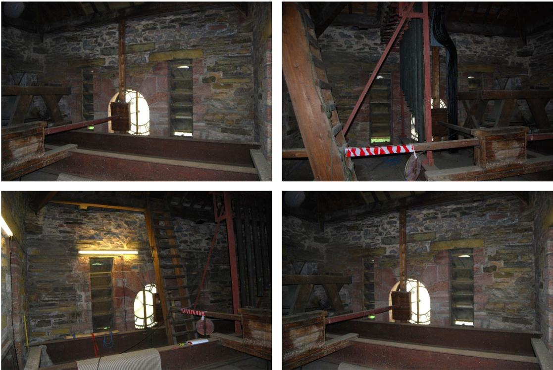
The walls at this level are of exposed stone masonry construction which has not been as heavily repointed as the clock chamber. The masonry appears to be in generally fair condition, consistent with its age, with no evidence of any significant cracking, recent or ongoing movement or other structural distress.
