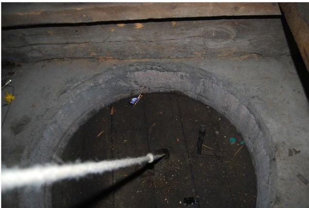
The trapdoor noted in the vaulted ceiling to the ground floor chamber is positioned below the clock case, severely limiting access.
