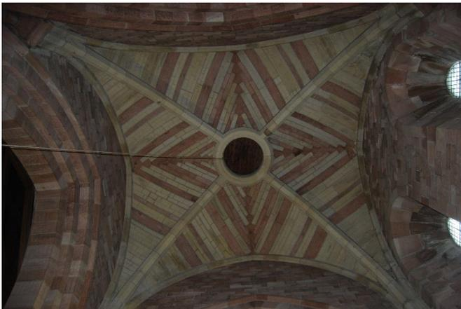
There is a vaulted stone ceiling to the ground floor chamber. This has a circular trapdoor in the centre to allow equipment to be hoisted up to the first intermediate chamber. Measurements from above showed that the trapdoor is approximately 1130mm clear diameter. Again, the masonry appears to be in generally fair condition, consistent with its age, with no evidence of any significant cracking, recent or ongoing movement or other structural distress.
