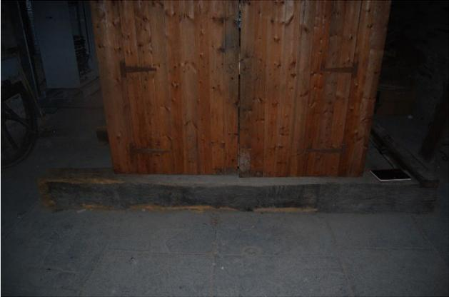
This chamber houses the clock mechanism, which stands in a wooden case and is supported on two timber spreader beams which run east west and bear onto a solid stone-flagged floor.
