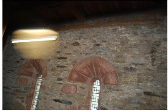
The walls at this level are of exposed stone masonry with rather heavy “butter” pointing. The masonry appears to be in generally fair condition, consistent with its age, with no evidence of any significant cracking, recent or ongoing movement or other structural distress.
