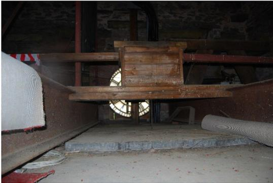
At present, the beams support a ring of nine tubular bells hung in a metal frame, a bell hung for static chiming in a timber frame and the clock drive linkage mechanism.
