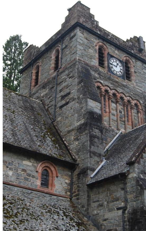
Just below parapet level, there is a continuous gutter, similar to that on the north elevation, which catches rainwater from the tower roof. This discharges via two downpipes to the north and south sides of the belfry louvre window opening onto the roof of the nave. The masonry appears to be in generally fair condition, consistent with its age, with no evidence of any significant cracking, recent or ongoing movement or other structural distress.
