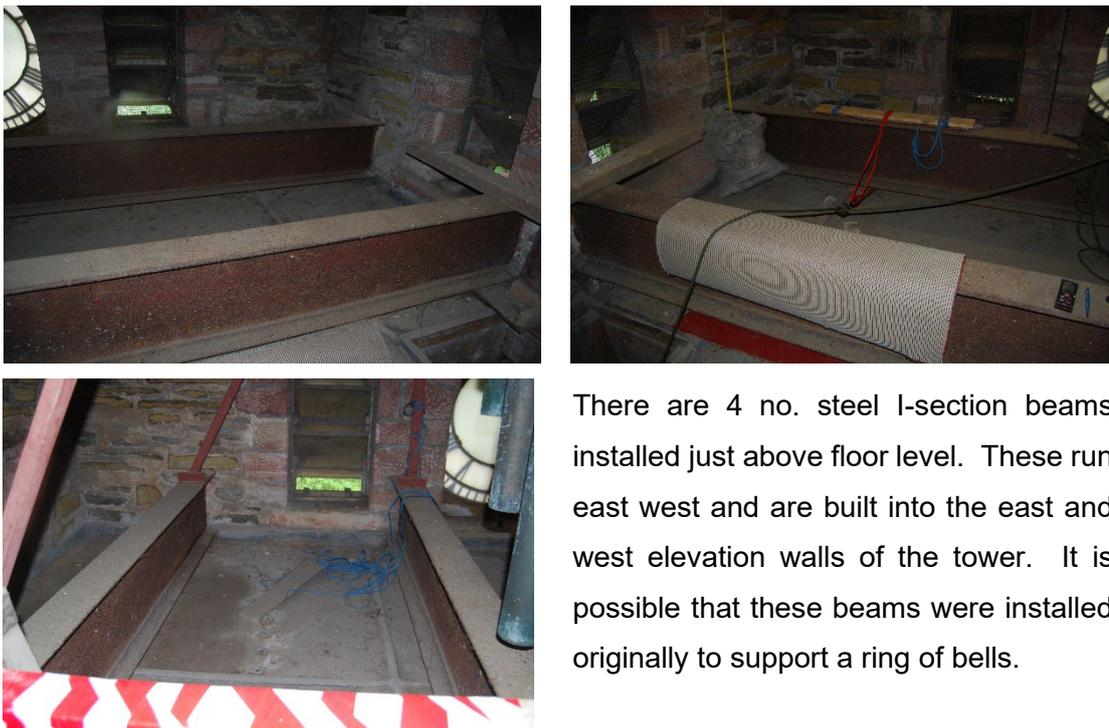
There are 4 no. steel I-section beams installed just above floor level. These run east west and are built into the east and west elevation walls of the tower. It is possible that these beams were installed originally to support a ring of bells.
