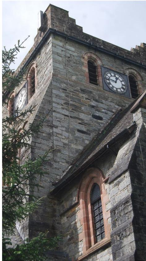
Just below parapet level, there is a continuous gutter, similar to that on the north elevation, which catches rainwater from the tower roof. The masonry appears to be in generally fair condition, consistent with its age, with no evidence of any significant cracking, recent or ongoing movement or other structural distress.
