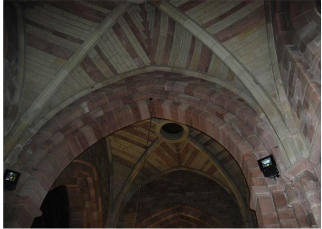
The walls at this level are of exposed stone masonry construction. There are almost full internal height archways in each elevation which take up almost the whole of the internal elevation widths, such that the tower is supported effectively by four substantial stone columns. The masonry appears to be in generally fair condition, consistent with its age, with no evidence of any significant cracking, recent or ongoing movement or other structural distress.
